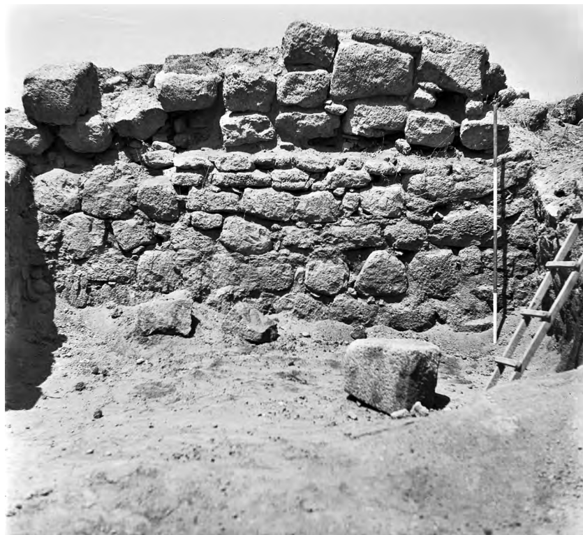
2. The northwestern wall of room E5, view from South-East.
