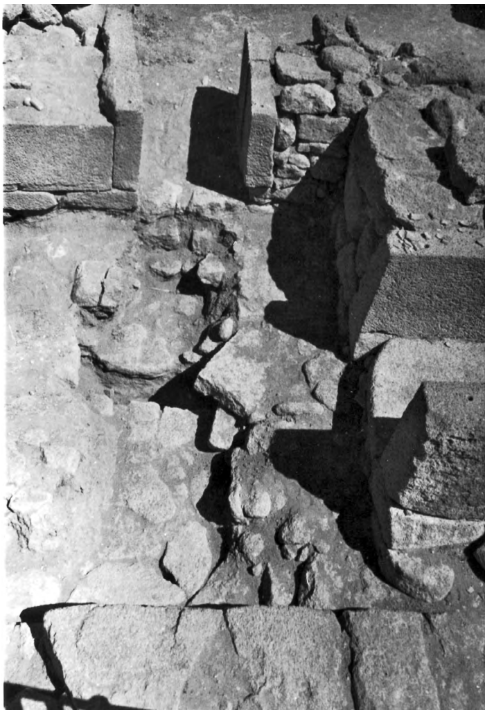
2. The drain between the staircases of Buildings A and B, view from South-West.
