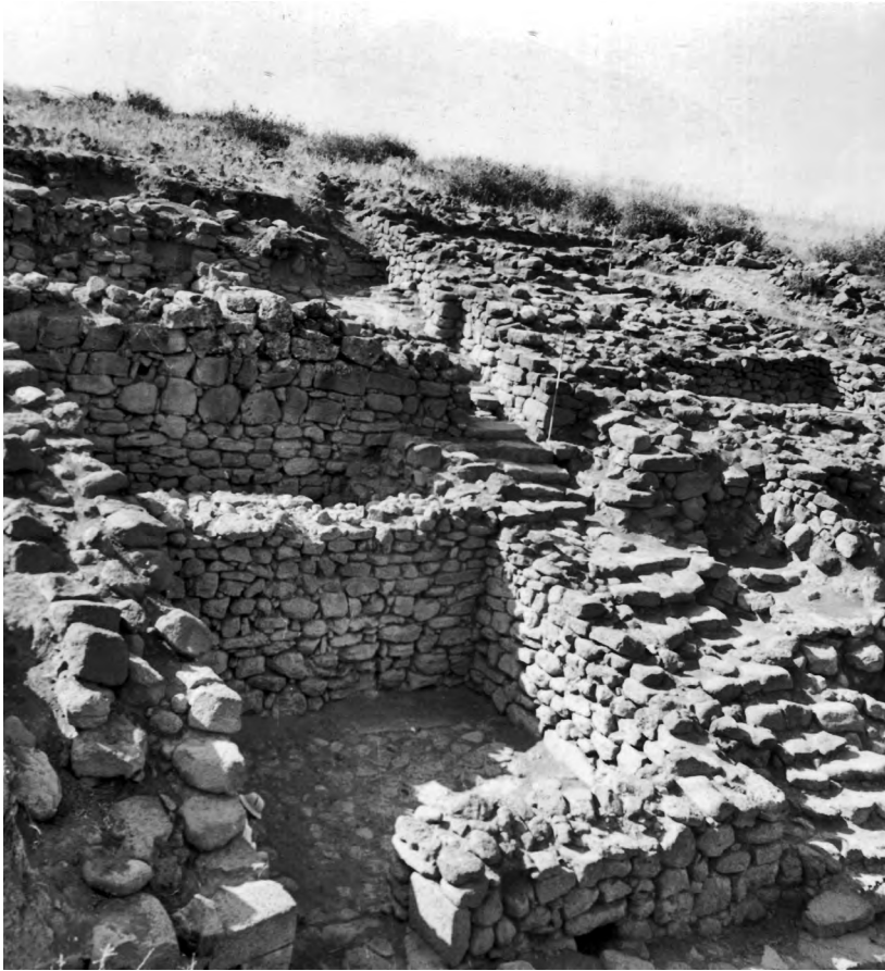
1. Gate K-5, view from South-East.
