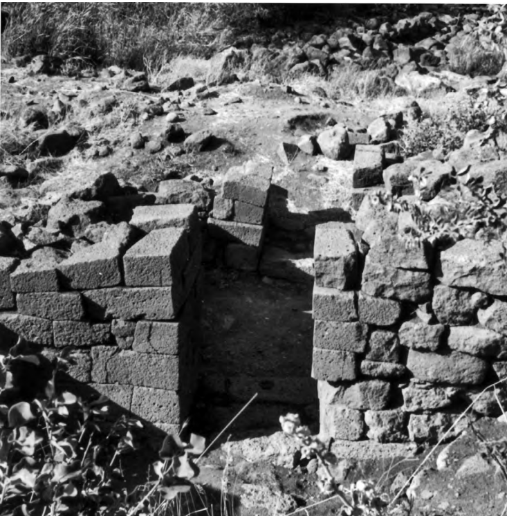
2. Another view of Gate K-2 from South.
