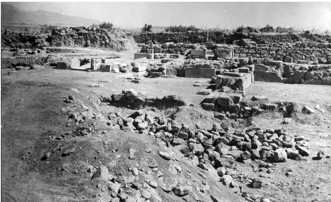
2. View of Building A from South.
