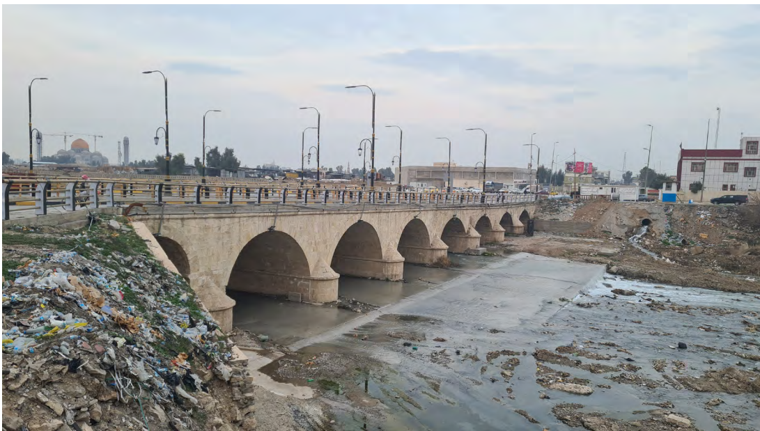
2. South side of lower Khosr bridge. View from south-west. Photograph January 2023.
