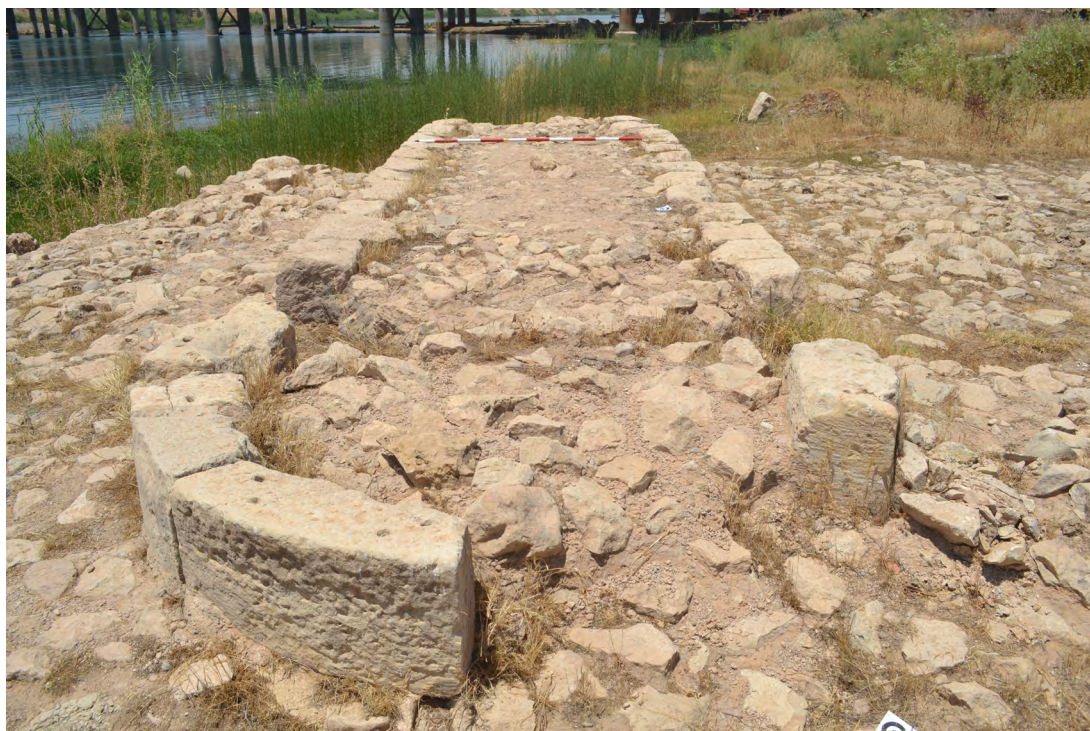
1. Pier 1 from south-east.
