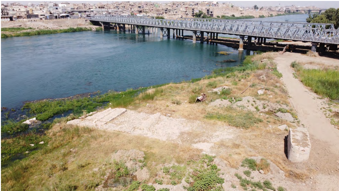
2. Remains of piers of the Old Bridge. View from south-east.
