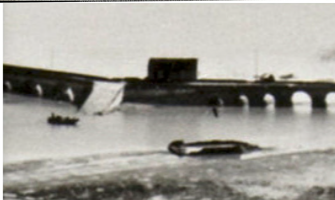
Above: Tigris flood-plain at Nineveh, with Nabi Yunus at top left, south-west corner of wall of Nineveh at top right, and Old Bridge, police post and lower Khosr bridge in centre. View from north-west. R.A.F. photograph CA 1206, dated 17 February 1919; below: enlargement of central features. Courtesy of the APAAME project (TNA Ref. CN 5/2 Part 4).
