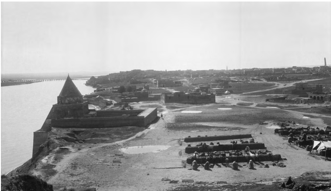
2. Distant view of Old Bridge before installation of New Bridge. Imam Yahya on left, with British cavalry(?) horses feeding. View from north-west, 1919-1920. Photograph N. 3658, probably taken by James Henry Breasted. ISAC Institute for the Study of Ancient Cultures, University of Chicago.
