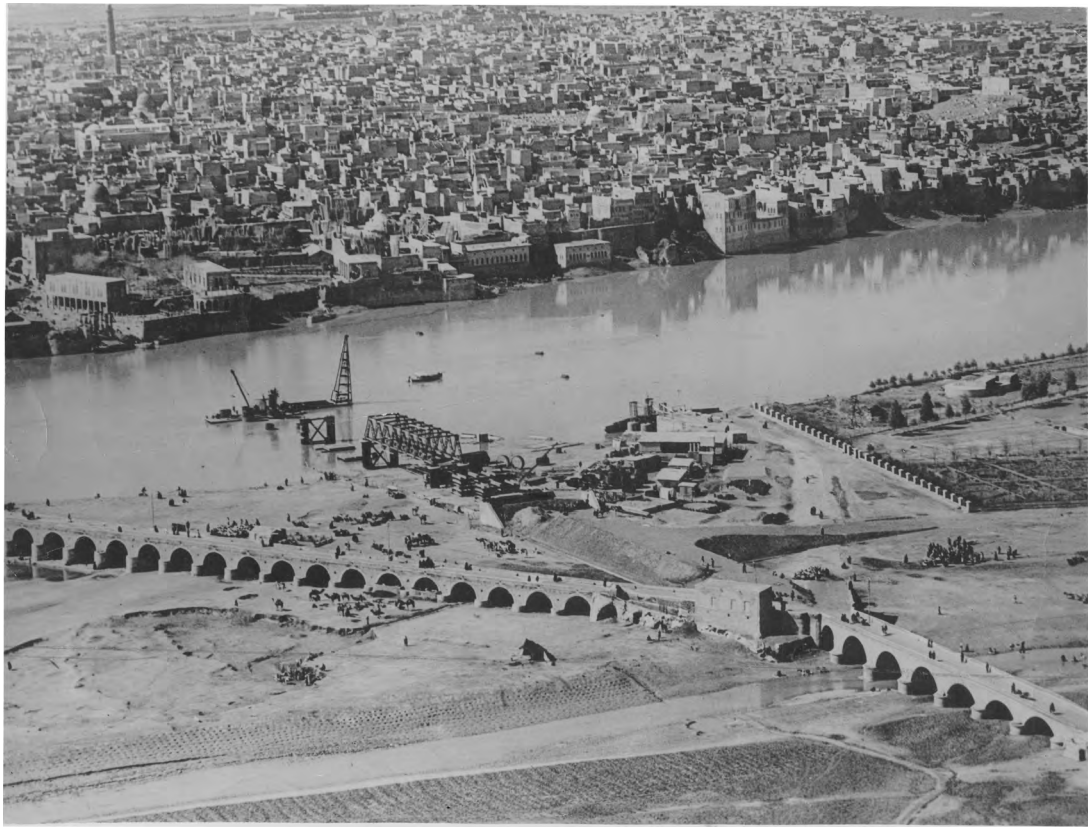
1. Mosul, with Old Bridge, Lower Khosr Bridge, and work in progress on Iron Bridge. View from east. R. A. F. photograph, c. 1932-3, stamped 8 October 1934. Courtesy Trustees of the British Museum.
