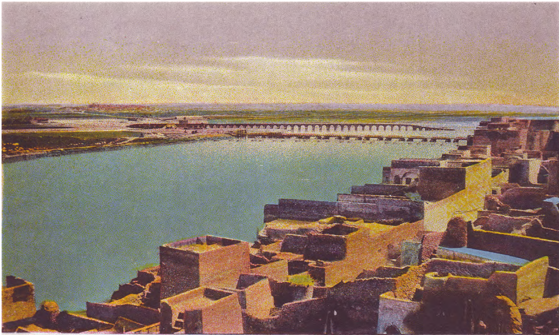
1. Distant view of breakwater pontoons, New Bridge and Old Bridge. View from north-west, 1919-1932. Postcard, Hasso Bros., Baghdad. Courtesy Trustees of the British Museum.
