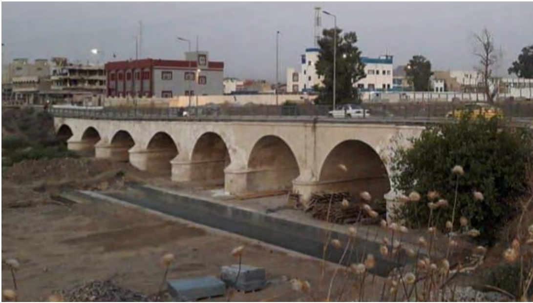
1. North side of lower Khosr bridge. View from west, c. 2022, Google Maps.
