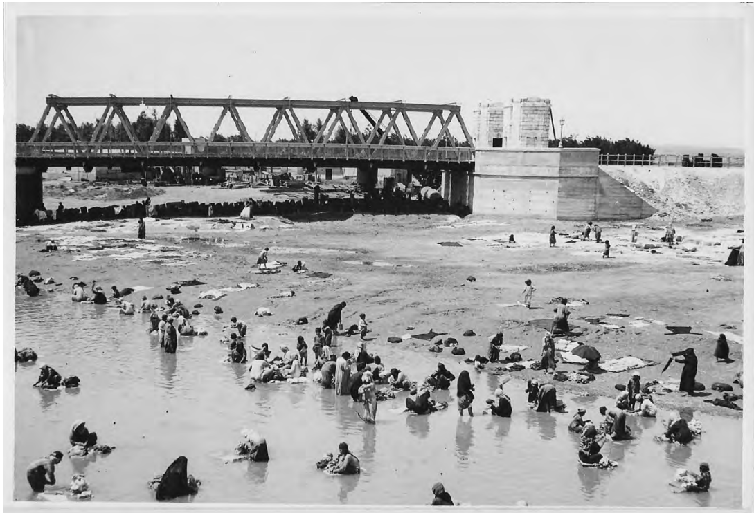
1. Iron Bridge during construction, with laundry in foreground. View from south, c. 1933. Donated by V. C. Ditchburn to the EAMENA project, School of Archaeology, University of Oxford.
