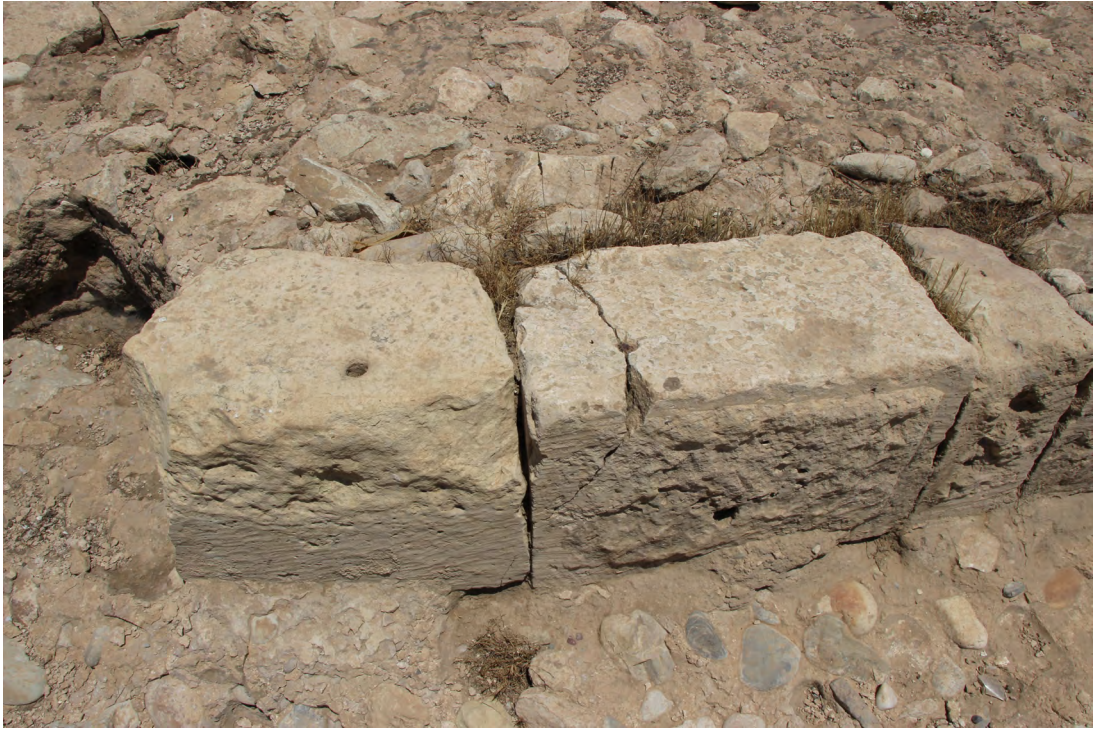
1. Iron rods anchoring the blocks of the first course to the ground: rusticated ashlar of Pier 1.
