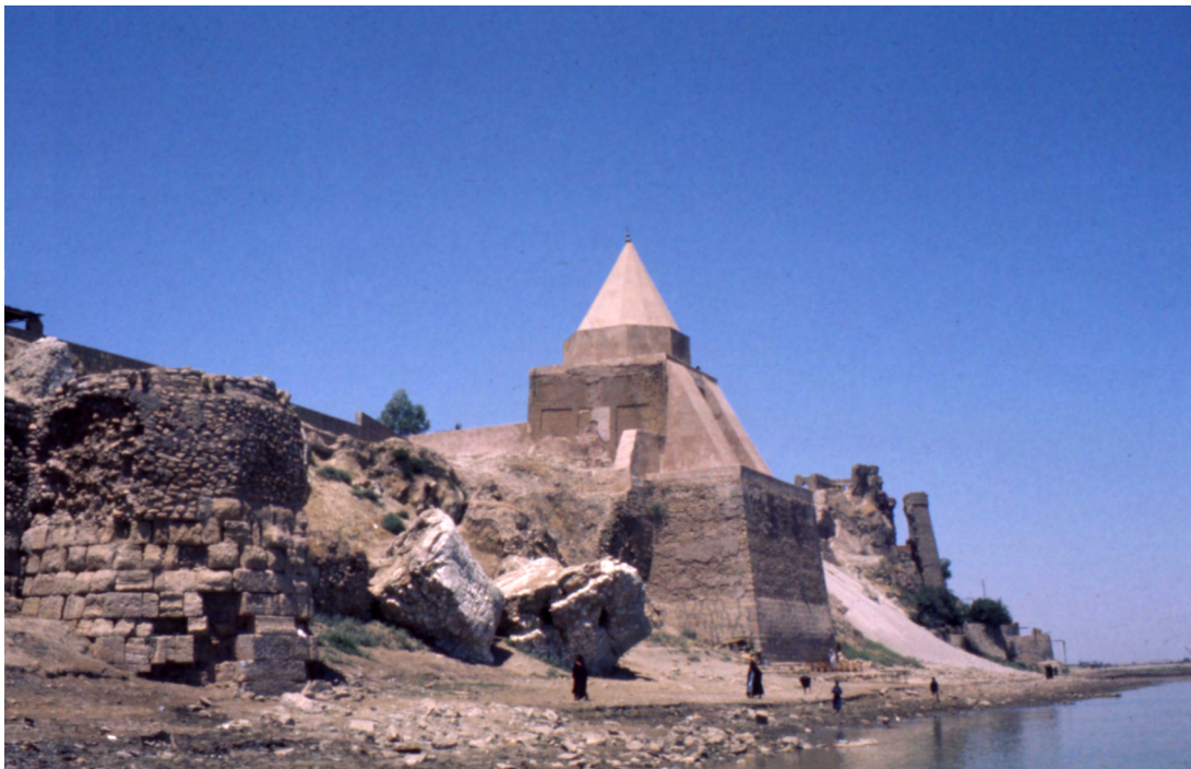
1. Right bank of Tigris at Mosul. From left to right: projecting stone tower of city-wall surmounted by successive phases, with Imam Yahya and Bash Tabia beyond. View from south-east. Photograph by J. E. Reade. Summer, 1965.
