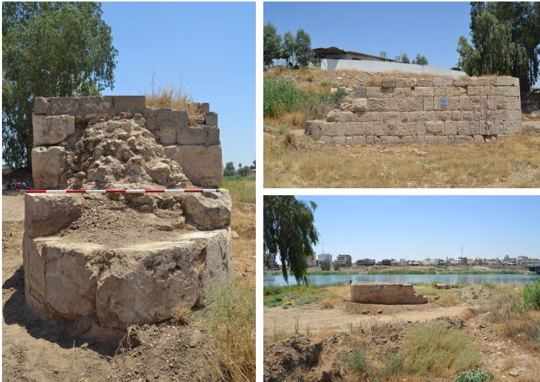
1. Pier 3. Left: view from north-west; right (above): view from west; right (below): view from east.
