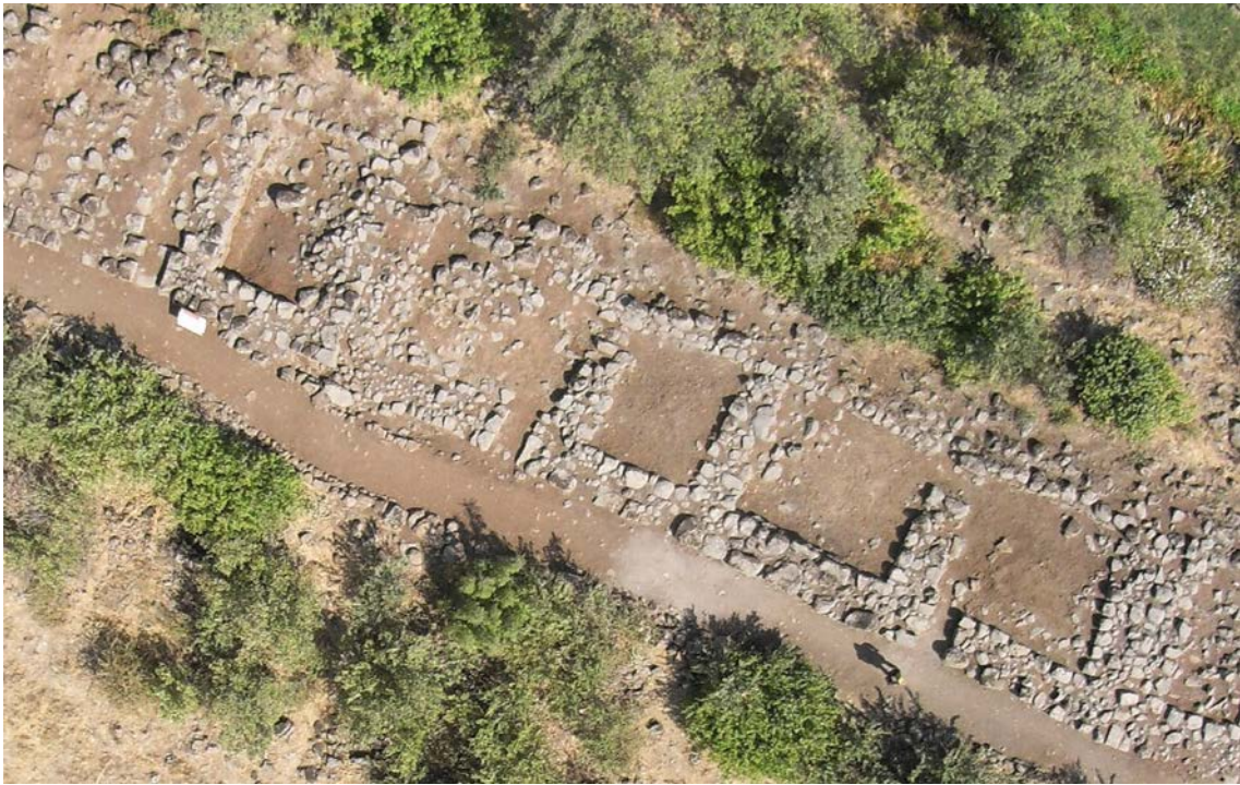
1. The northern casemates. Aerial view of CN 6 – on the right – and CN7 – on the left, in 2008.
