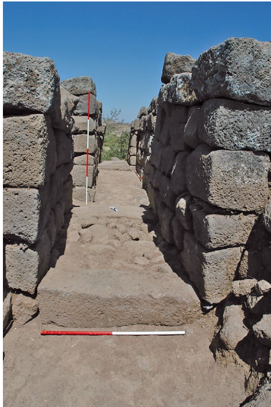
1. The adjoining casemates south+ and, in background, the fortress P, from the south. The wall W.1605 is visible in the middle of the photo. The first meter indicates the possible access to the casemate.
