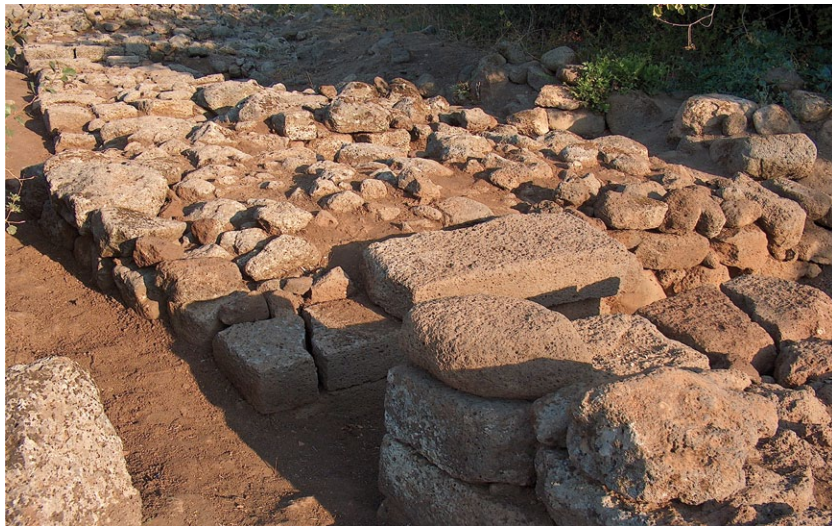
2. The northern casemates. Detail of the access to CN2 from SE. State of preservation of the structure in 2008.
