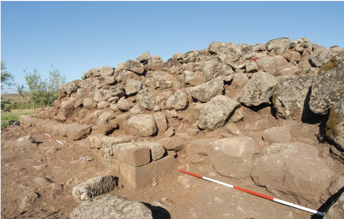
1. The fortress P. The western wall W.1611. The southern edge of the wall, and the connection with the adjoining casemate south, from the SW.
