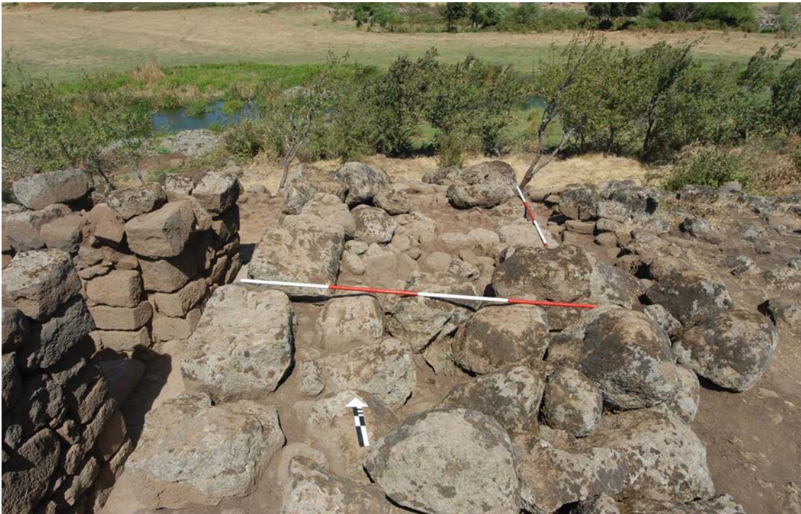
1. The fortress P. The northern wall W.1609 from the south. Some remains of the adjoining casemates east are visible on the right.
