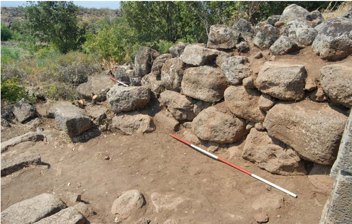
1. The western sector of the gate K-3 in a photo taken during the restoration season in 2008. The inner chamber L.807 from the SE. Detail of the walls W.805, on the right, and W.830, on the left.
