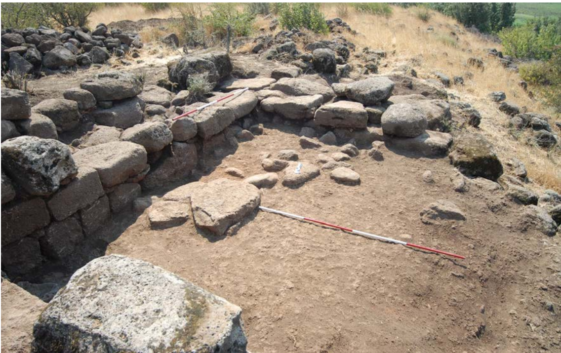
2. The building P2. The eastern part of the room L.1627 and the sparse remains of the floor. The western part of the room has been washed away.
