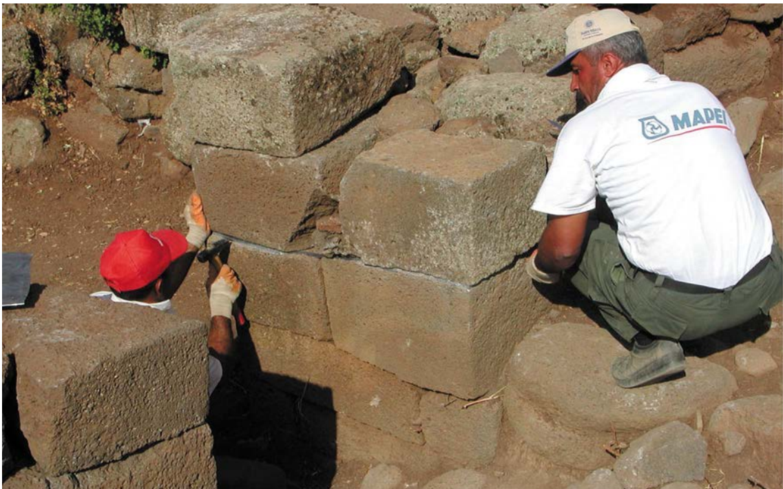
2. The area K-3. The restoration of the pier W.804 in 2008.
