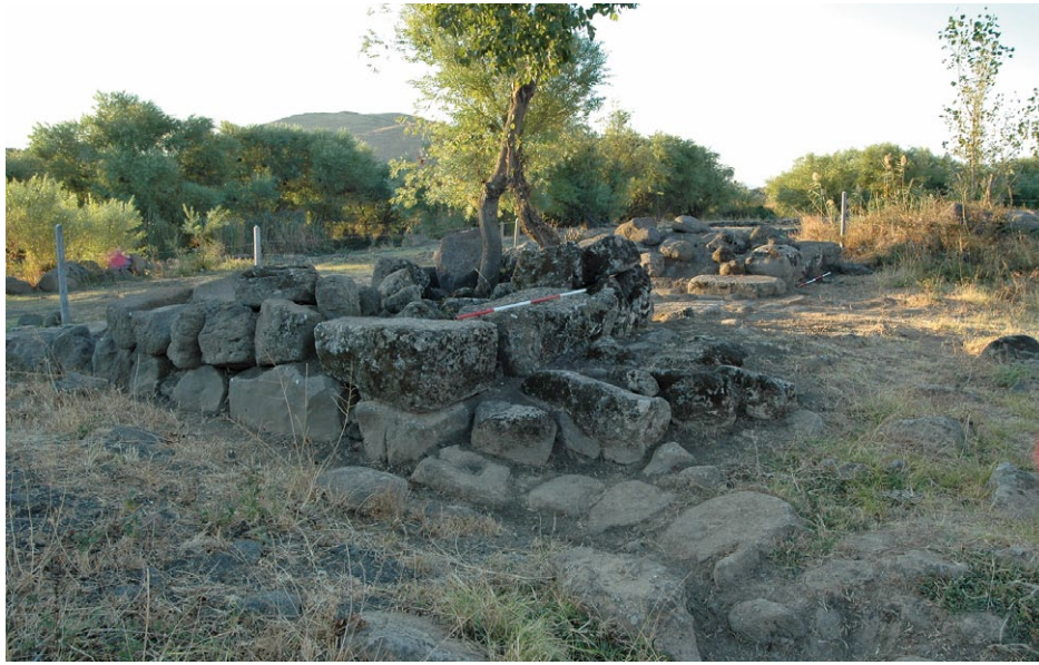
1. The northern tower of the gate K-6. State of the structure in 2005.
