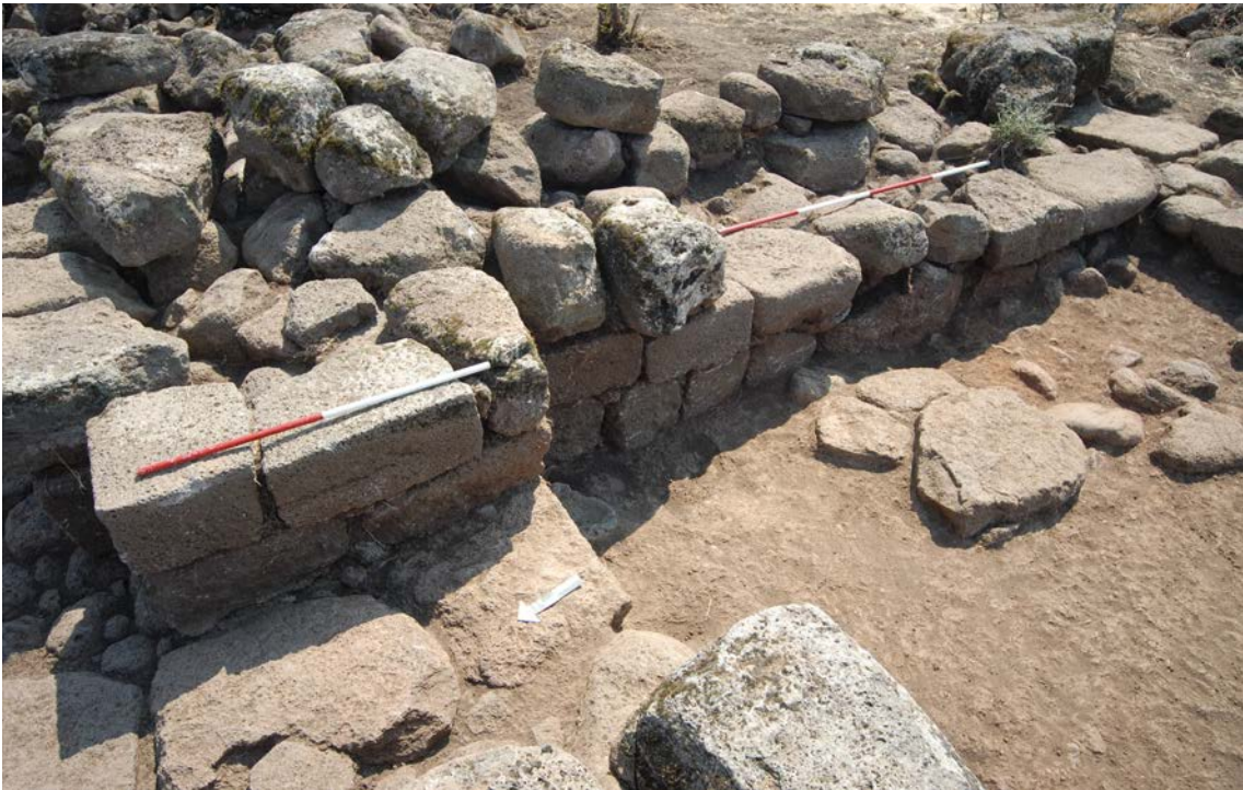
1. The building P2. The gateway L.1618 and the southern pier of the passage, from the west. The eastern part of the room L.1627 is visible on the right.
