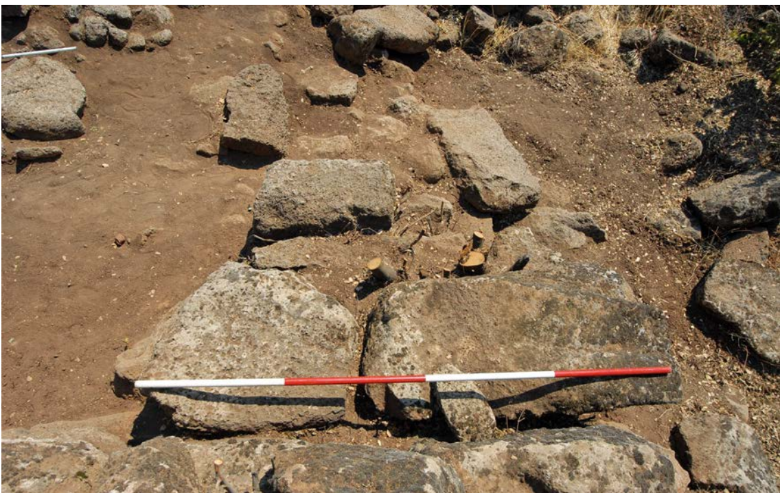
2. The western sector of the gate K-3 in a photo taken during the restoration season in 2008. A detail of the massive, outer wall of the gate, W.830, from the north.
