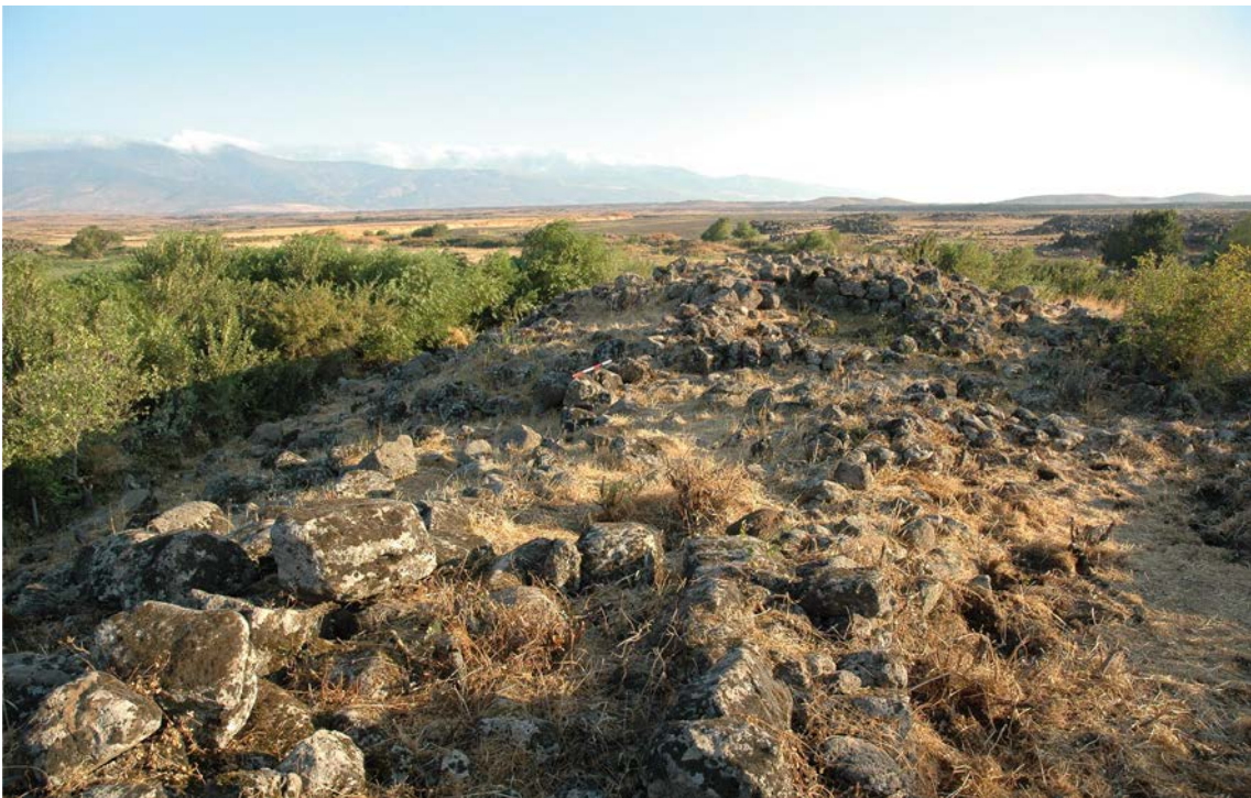
2. The area P. The state of preservation of the structures above the surface before excavations in August 2006. A view of the adjoining casemates south and of fortress P from the south, from the building P2.
