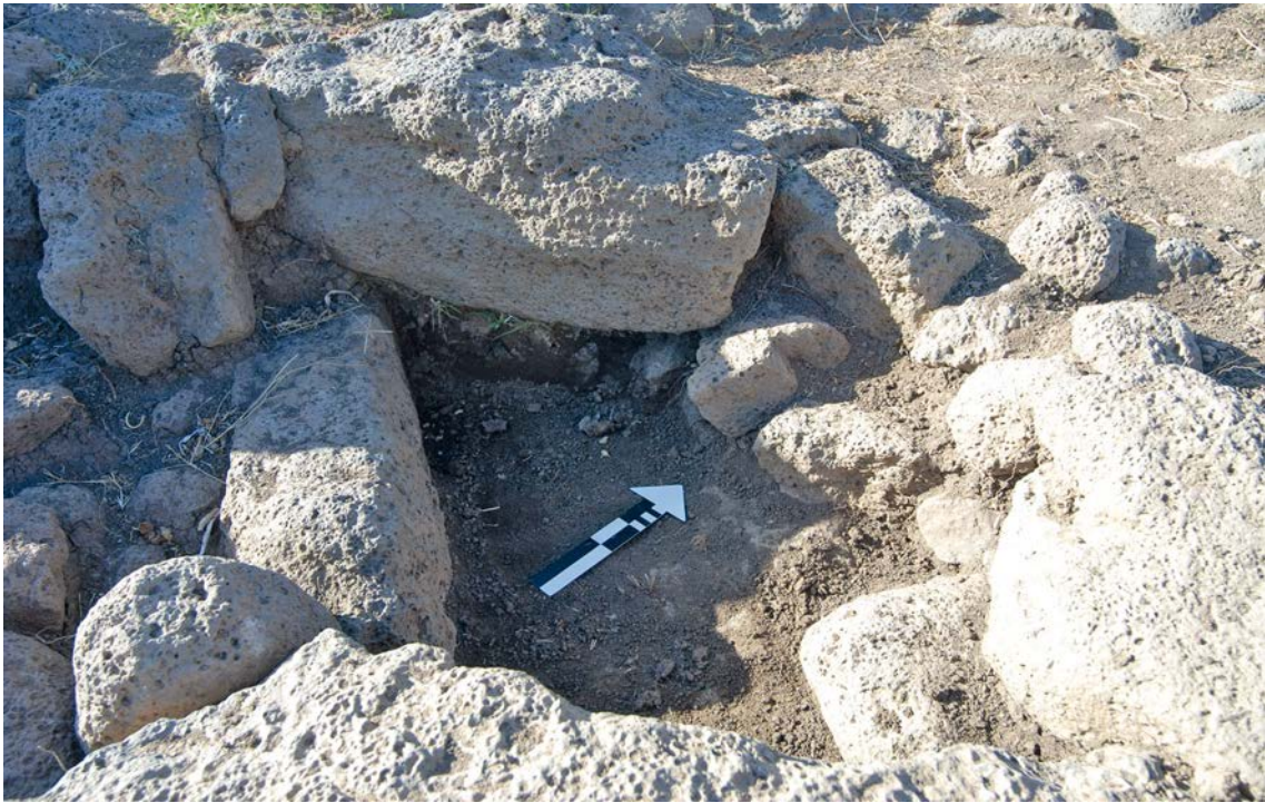
1. The gate K-1. A detail of the section of the drain D.1028 exposed in the passage L.1013, from the SE.
