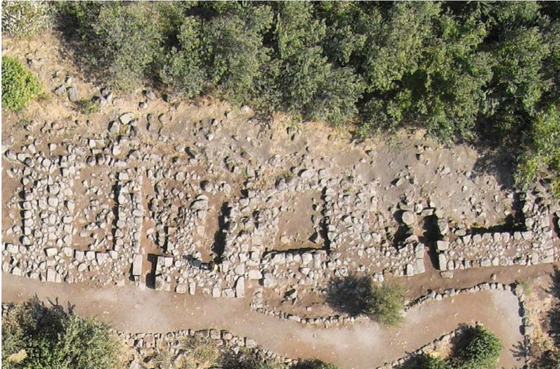
1. Aerial view of a section of the northern casemates: CN3, CN4 and CN5 are visible from right to left.
