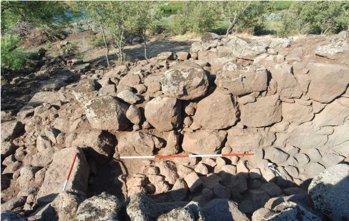
1. The fortress P. Detail of the southern façade of the wall W.1634, from the SW.
