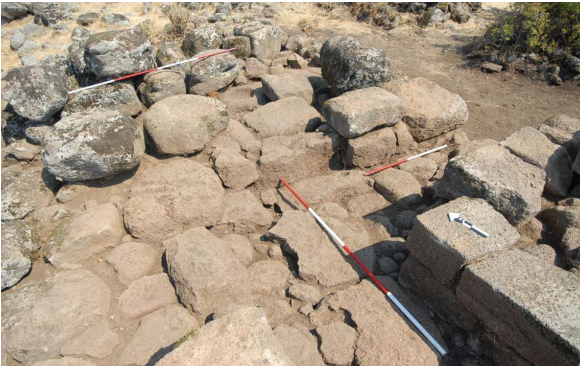
2. The building P2. Detail of the wall W.1615, with the niche of the door socket, from the SW.
