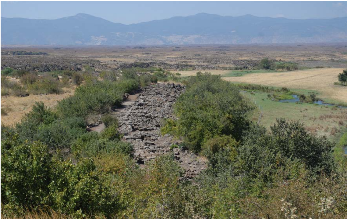
1. The northern sector of the lower town fortification wall. The northern casemates, from the east, from the upper town. The structures visible on the surface in 2008, and the rich vegetation.
